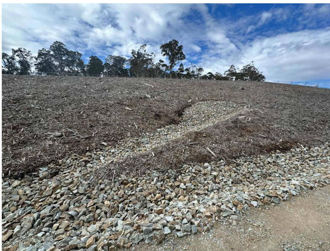
Plate 16: Erosion and sediment controls installed to address water seepage issues and prevent soil loss at Maragle Switchyard – Project West (Inspection date 10/09/2025)
