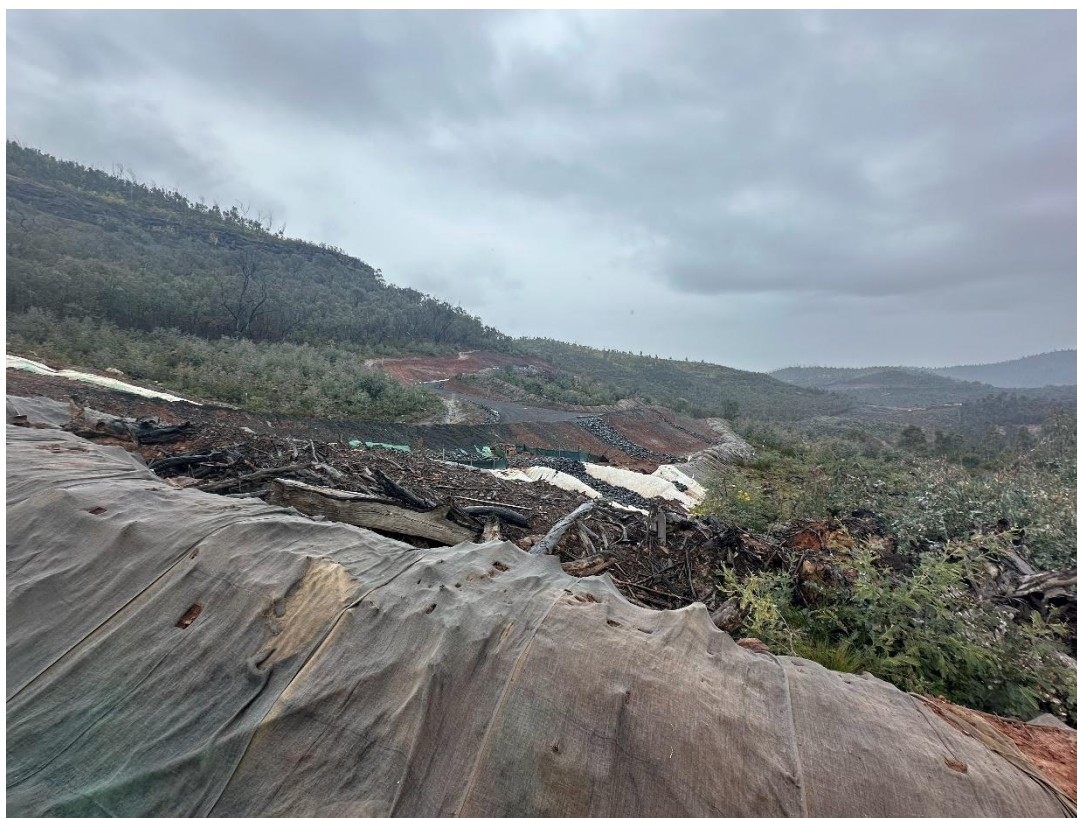
Plate 18: Degraded geofabric on some of the batters along Track 8 – Project East (Inspection date 10/09/2025)
