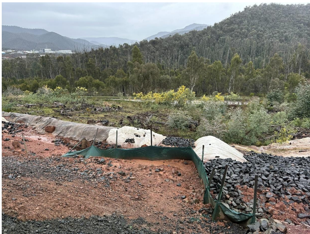
Plate 17: Fallen sediment fence on Track 8 – Project East (Inspection date 10/09/2025)
