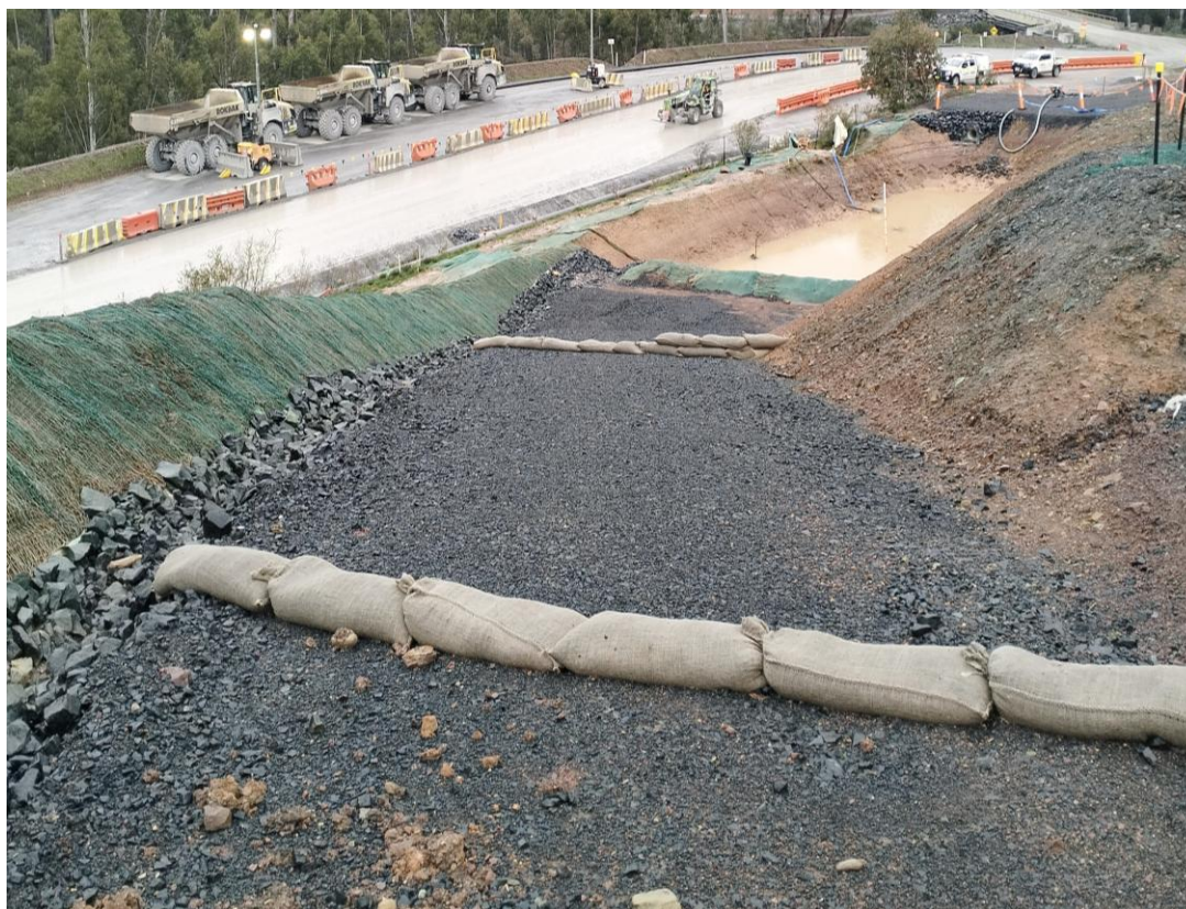
Plate 13: Erosion and sediment controls leading to sediment basin along Track 8 – Project East (Inspection date 10/09/2025)
