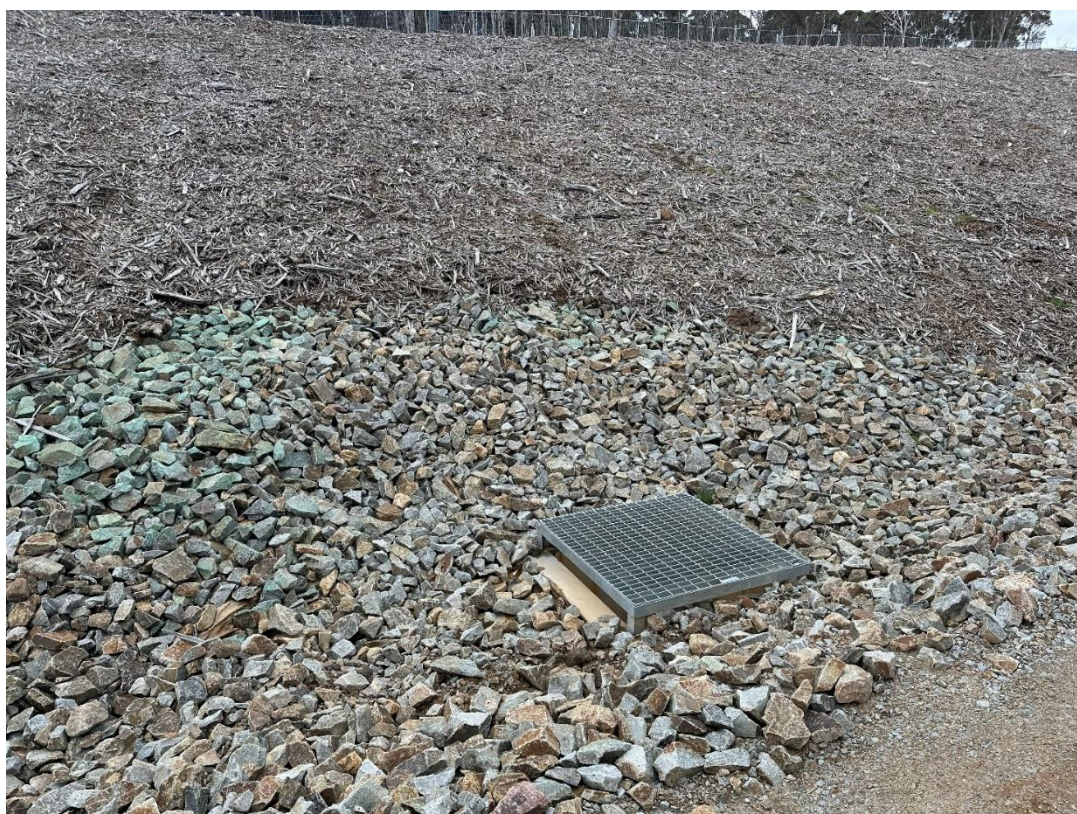
Plate 24: Erosion and sediment controls well maintained and effective - Maragle Switchyard (Inspection date 09/09/2025)
