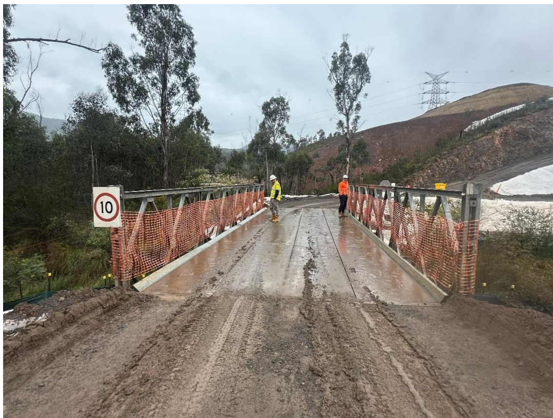
Plate 21: Temporary Sheep Station Creek Bridge deck clear of sediment - Project East (Inspection date 10/09/2025)
