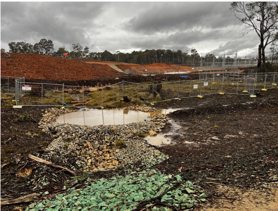
Plate 12: Installed erosion and sediment controls around the “Duck Pond” looking towards the 500 kV substation sediment basin (Inspection date 10/09/2025)
