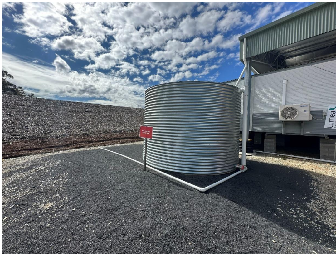
Plate 23: Fire tank full and correctly signposted - Maragle Project Construction Compound (Inspection date 09/09/2025)
