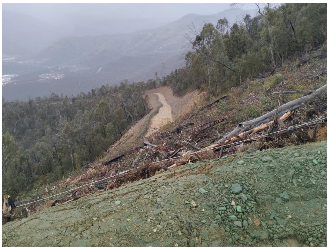
Plate 14: Erosion and sediment controls and soil binder installed along Track 5 (as viewed from Pad 10) – Project East (Inspection date 10/09/2025)
