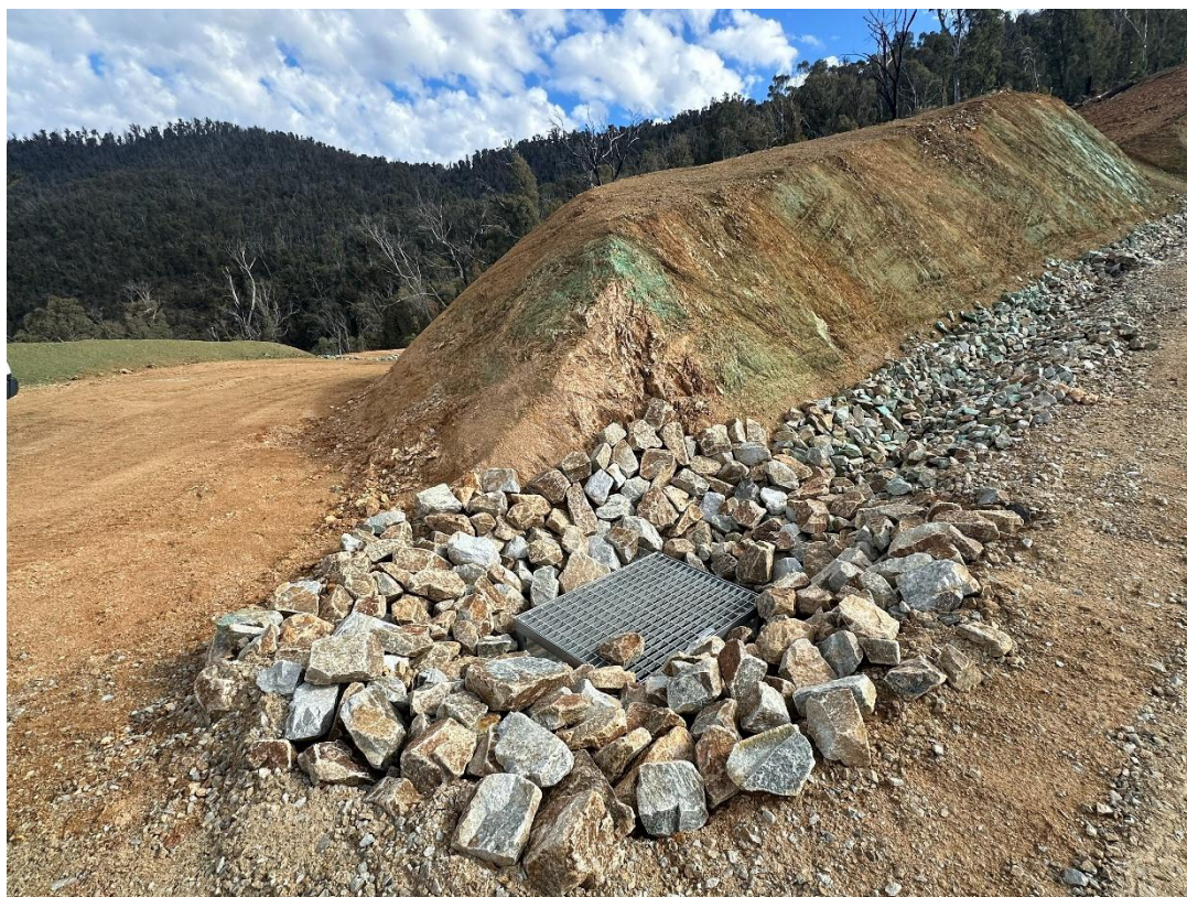
Plate 15: Installed erosion and sediment controls on Track 2 (Inspection date 10/09/2025)
