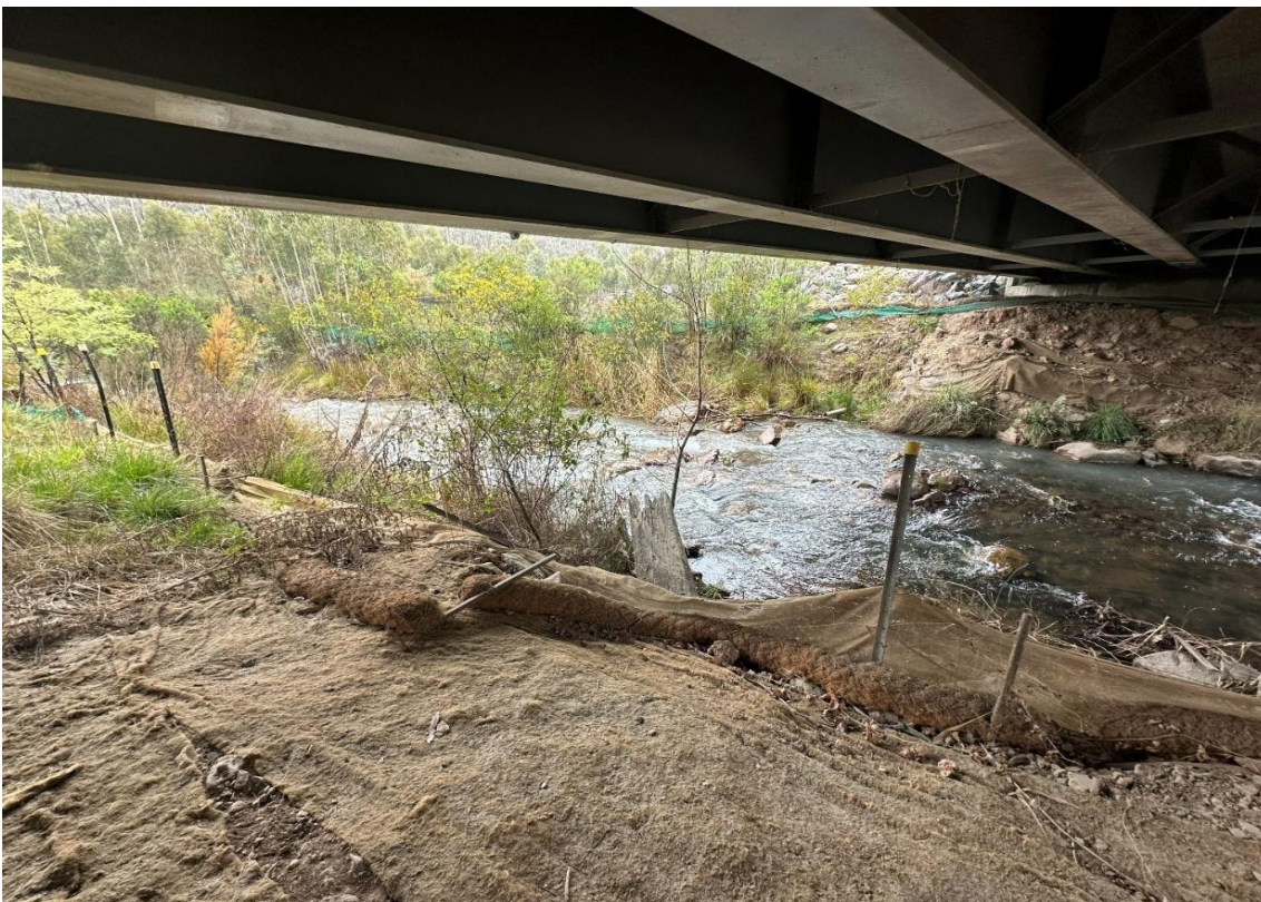
Plate 30: Ineffective erosion and sediment controls located on edge of Wallace Creek - Project East (Inspection date 10/09/2025)
