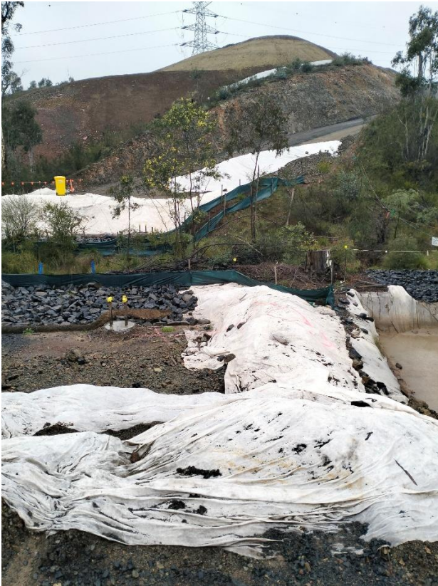
Plate 19: Implementation of erosion and sediment controls around the temporary Sheep Station Creek Bridge – Project East (Inspection date 10/09/2025)
