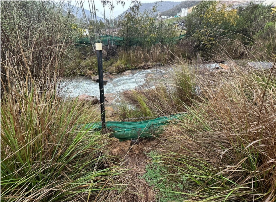
Plate 31: Erosion and sediment controls located on edge of Wallace Creek. Sediment fences were observed not embedded – Project East (Inspection date 10/09/2025)
