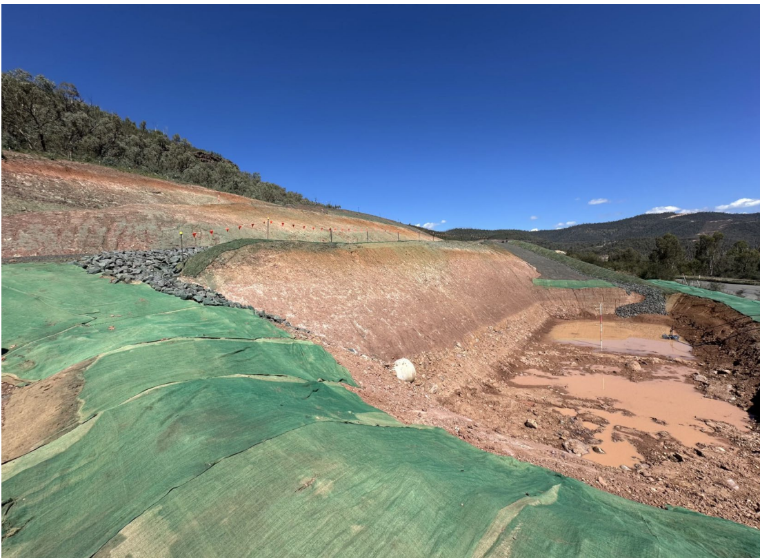
Plate 22: Sediment basin located near the base of Track 8 (Inspection Date: 12/03/2025).
