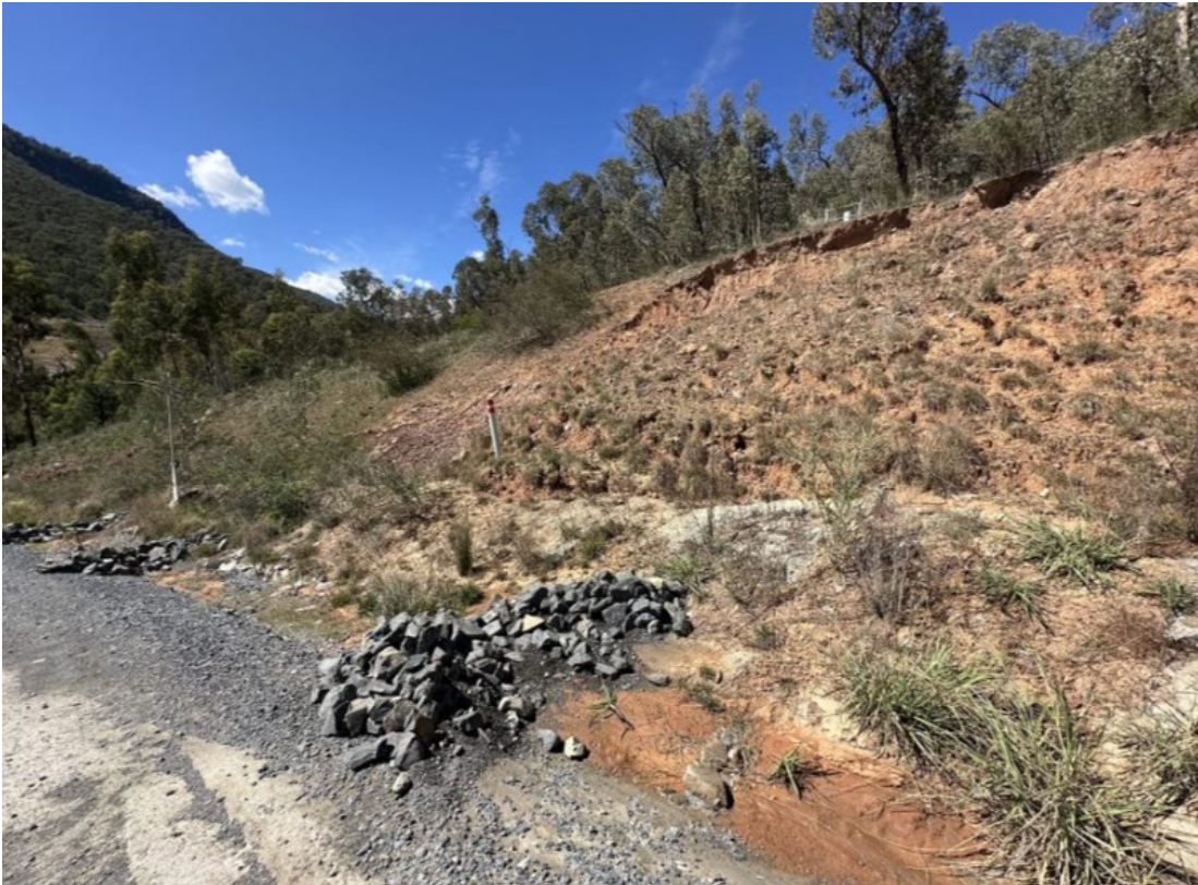
Plate 43: Dirty water diversion with rock checks located on Track 8 (Inspection Date: 12/03/2025).
