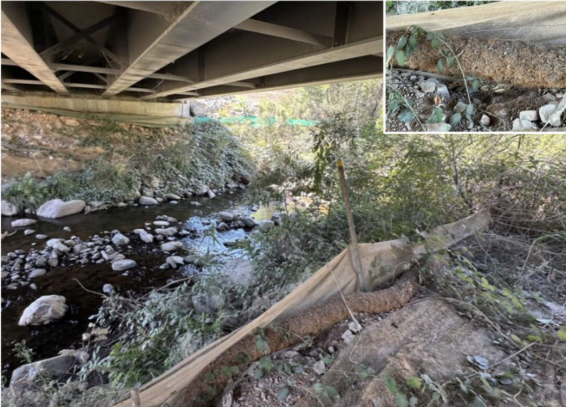
Plate 21: Erosion and sediment controls located on edge of Wallace Creek. Sediment fences were observed not embedded (Inspection Date: 12/03/2025).
