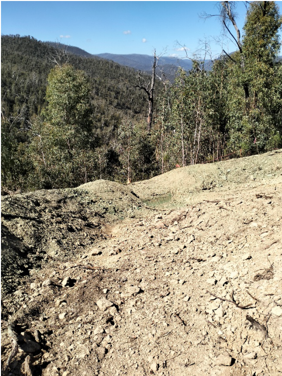
Plate 27: Track 4 Sediment trap, evidence of soil binder present however outlet is unlined (Inspection Date: 12/03/2025).
