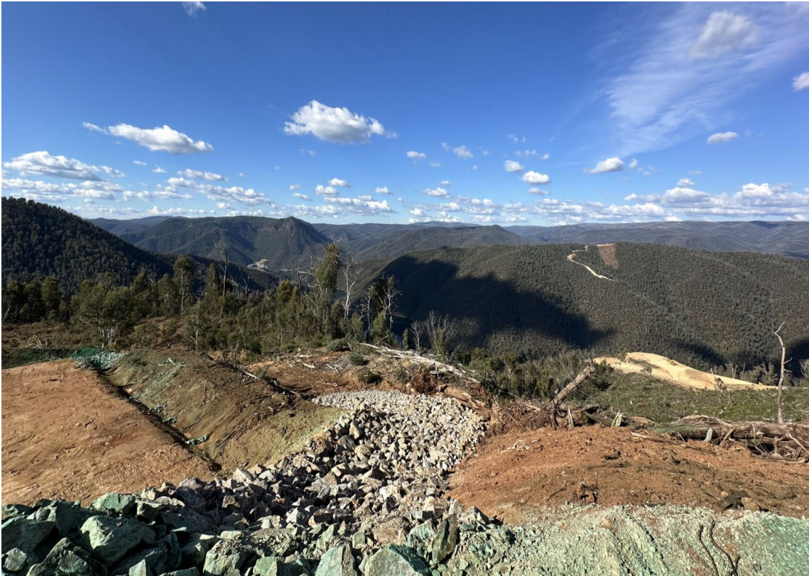
Plate 23: Rock drains located along the western alignment (Inspection Date: 12/03/2025).
