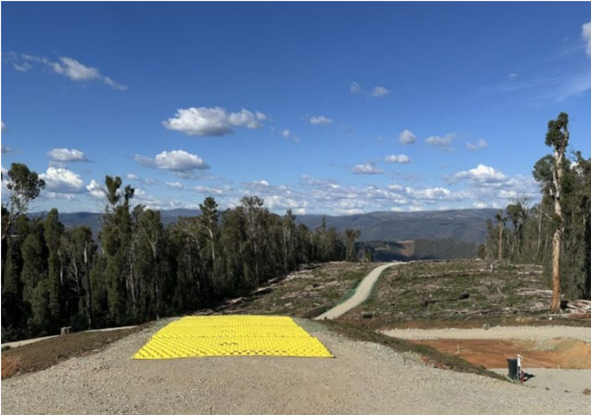
Plate 35: Rumble girds installed at the entrance and exit of Track 10 (Inspection Date: 12/03/2025).
