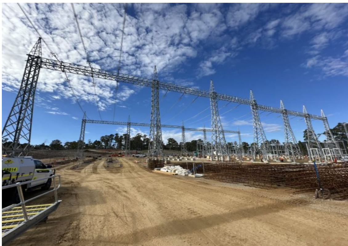
Plate 31: Overview of multiple gantries constructed at the Maragle Substation Project Area (Inspection Date: 13/03/2025).
