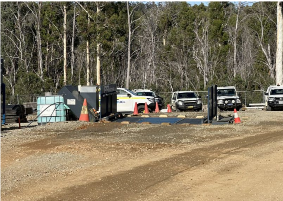
Plate 34: Wheel washing station located within the Maragle Project Construction Compound (Inspection Date: 13/03/2025).
