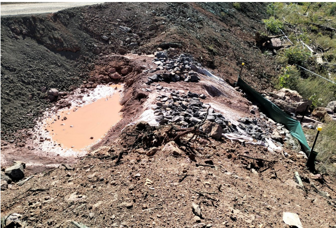
Plate 28: Track 5 Sediment Trap with evidence of sediment overflow in outlet (Inspection Date: 12/03/2025).
