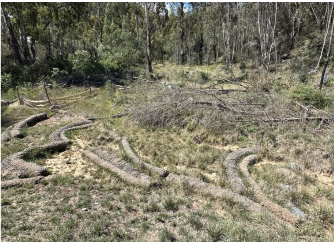
Plate 20: Erosion and sediment controls leading into Wallaces Creek (Inspection Date: 12/03/2025).
