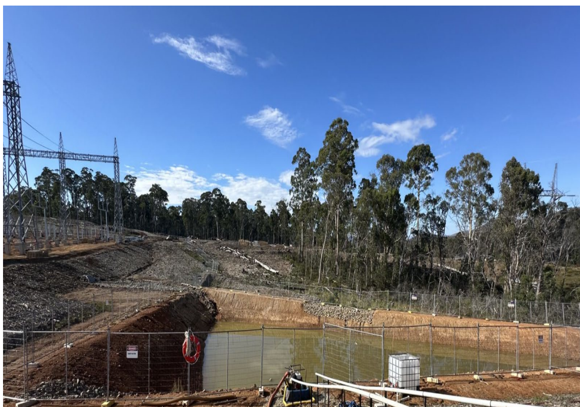
Plate 30: Sediment basin at the Maragle Project Construction Compound (Inspection Date: 12/03/2025).
