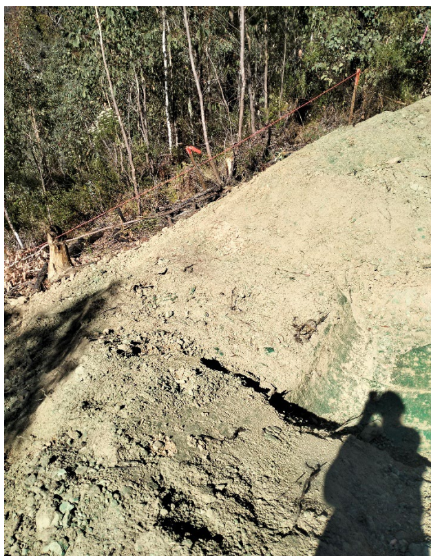
Plate 26: Track 4 Sediment trap, evidence of soil binder present however outlet is unlined (Inspection Date: 12/03/2025).
