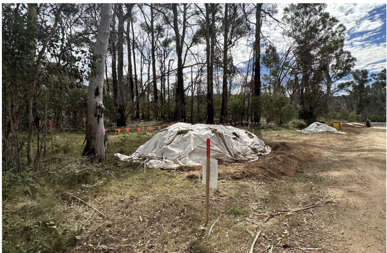
Plate 12: Stockpile controls in use located near Elliott Way/Access Track South Intersection (12/03/2024)
