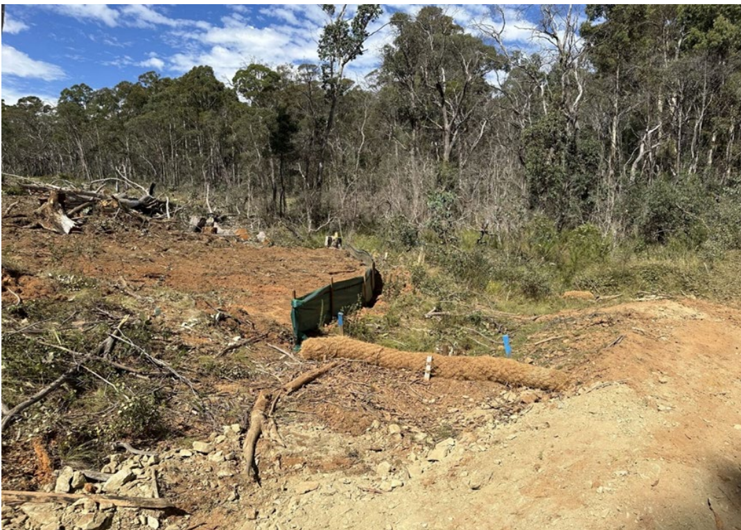
Plate 8: Sediment and erosion controls located towards the edge of the clearing extent at Maragle Substation Project Area (12/03/2024)
