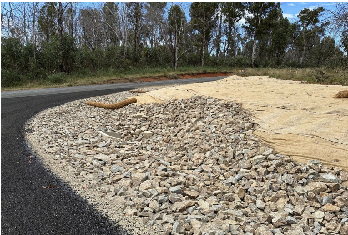
Plate 6: Rock banks, cogs and culvert installed alongside Elliott Way/Access Track South Intersection (12/03/2024)
