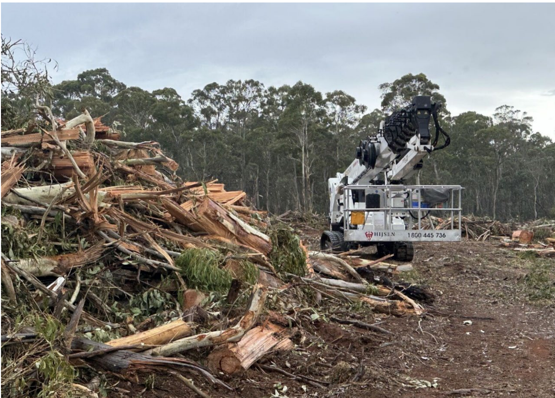
Plate 14: Equipment used to assist in pre-clearing e.g. Spider Boom located within Maragle Substation Project Area (14/03/2024)
