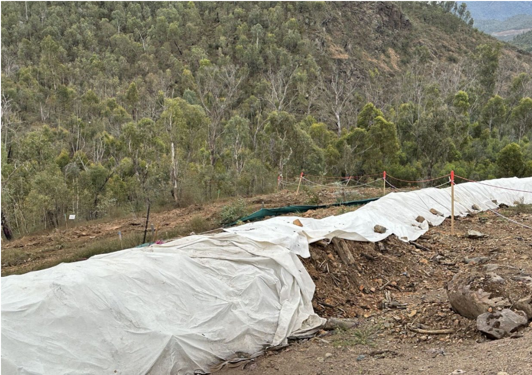
Plate 9: Erosion and sediment controls located at Lobbs Hole Project Compound (14/03/2024).
