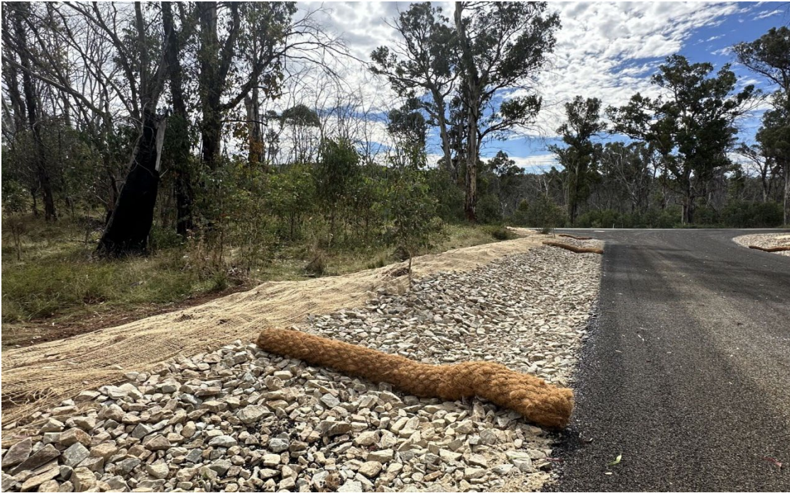
Plate 5: Rock banks and cogs installed alongside Elliott Way/Access Track South Intersection (12/03/2024)
