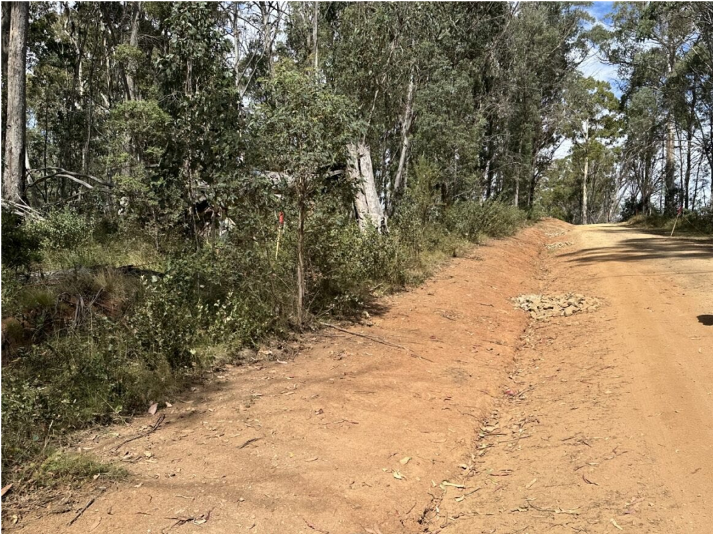
Plate 7: Rock drain check and diversion drains located within Maragle Substation Project Area (12/03/2024)
