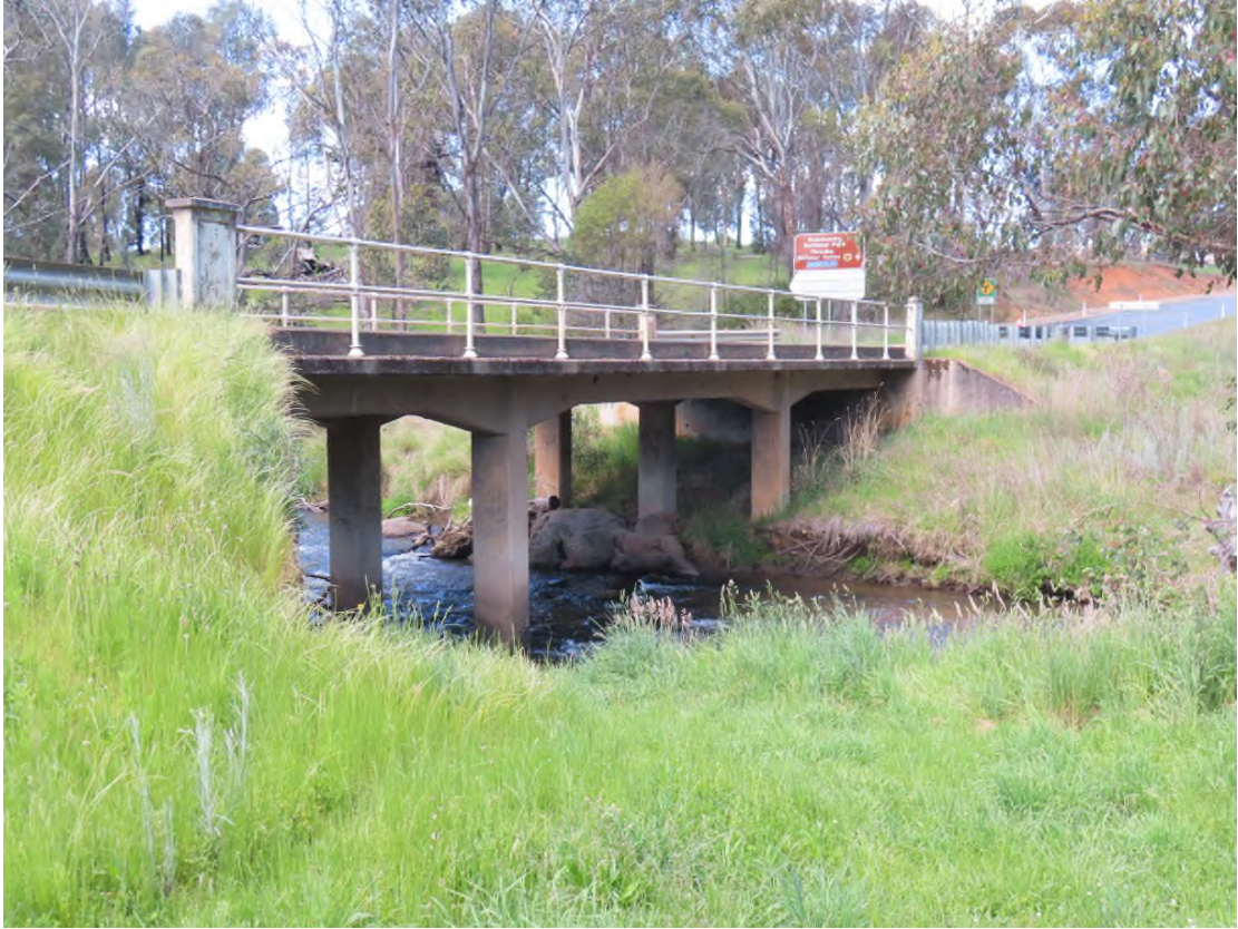
Photo 9. South side view of bridge.
