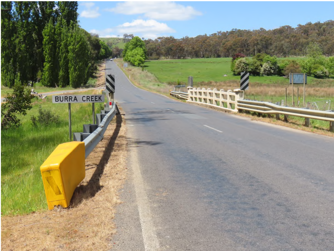
Photo 2. View of bridge from west end.
