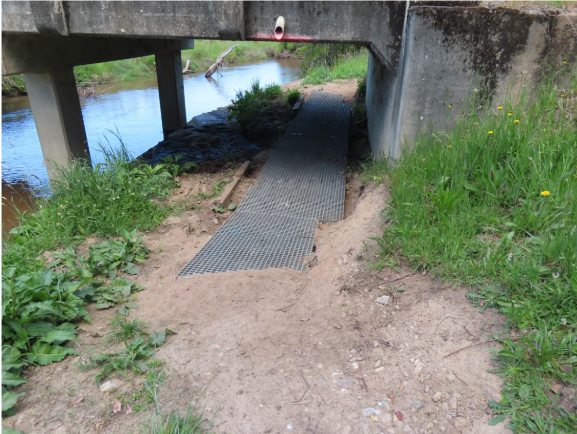
Photo 7. Track of composite mesh material under Tumbarumba abutment.
