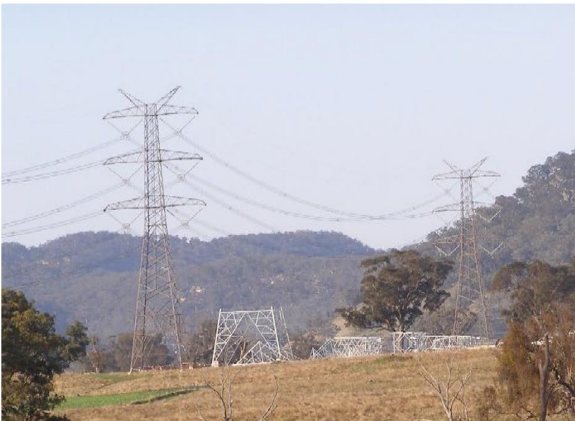
Figure 5-6: Pre-dulled towers with a galvanised tower under construction adjacent. The photograph illustrates the shine and potential reflection of a standard tower without treatment. Image source: Supplementary Landscape and Visual Impact Assessment Rev 01 prepared by Landform Architects March 2022
