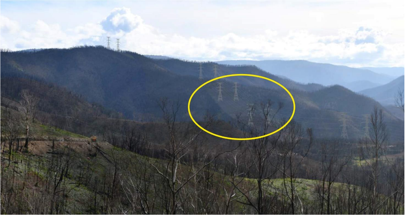
Figure 5-3: Visual simulation of lattice towers to be painted olive green to help make them recede into the background. The towers to the top left are 10L & 10R and run down to 6L & 6R. The only two pairs in this photo simulation which will be painted olive green will be pairs 7 and 8 (in yellow circle) as they have more of a vegetative background. The other 3 sets of towers 6,9 & 10 will have a dull grey treatment as their background has been assessed as predominantly visible against the sky. Lobs Hole Ravine Road indicative viewpoint. Image source: Landscape Character and Visual Impact Assessment Rev 04 prepared by Jacobs December 2020
