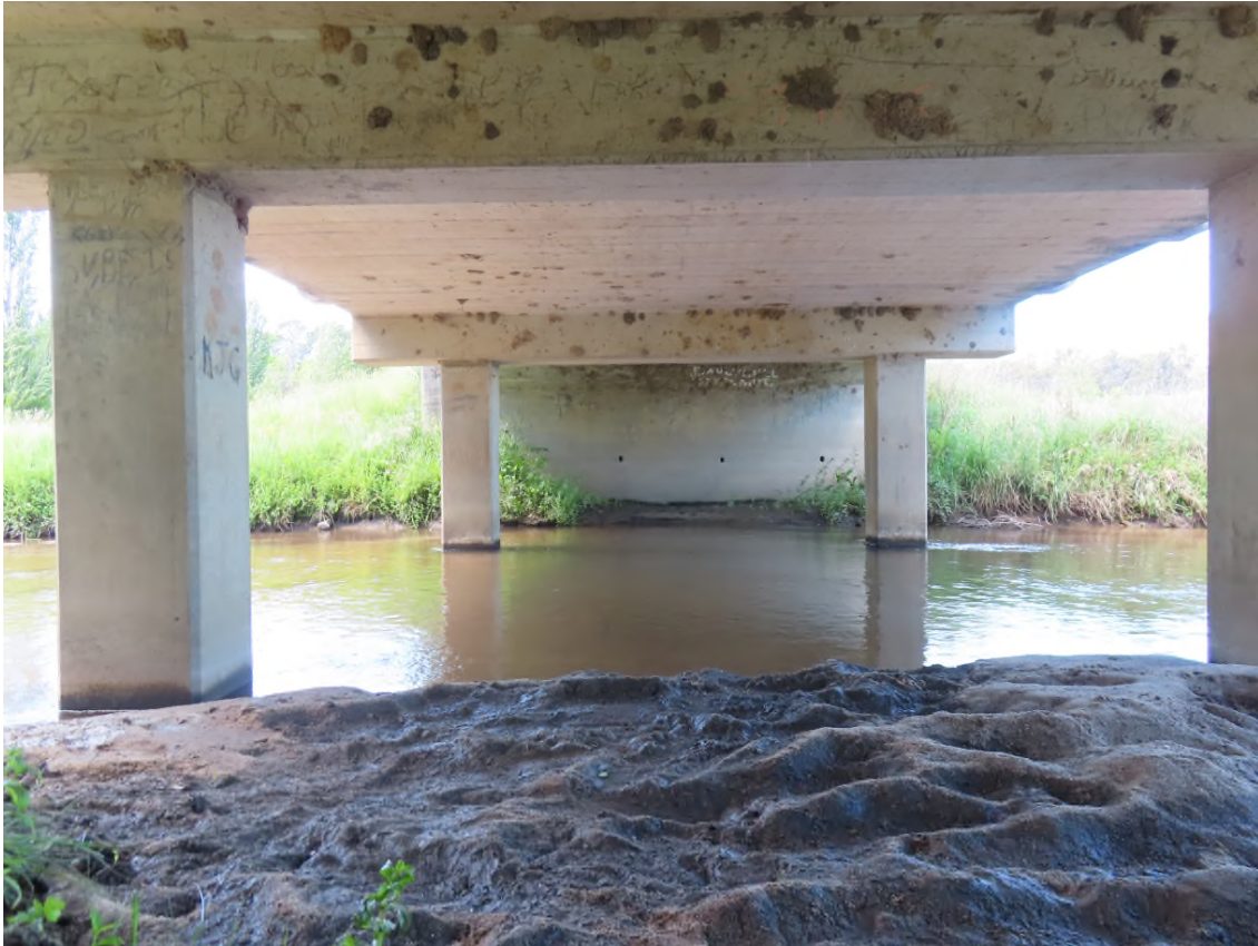
Photo 3. Underside of deck with pier columns and headstock. West span.
