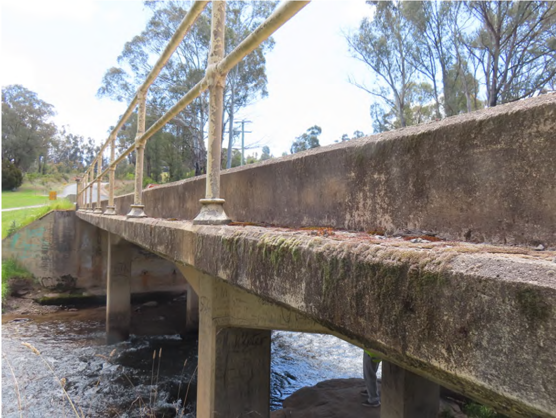
Photo 21. Side of bridge showing fixing arrangement for bridge railing.
