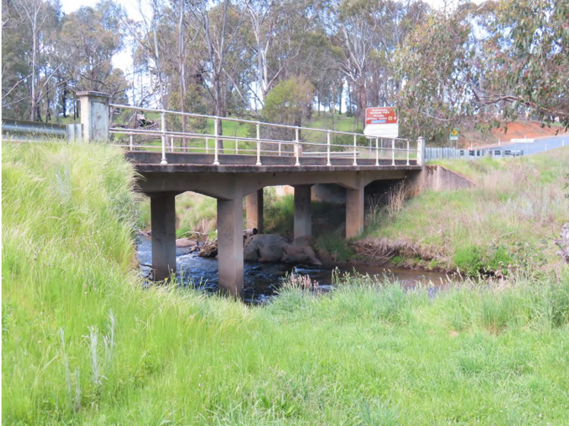
Photo 9. South side view of bridge.
