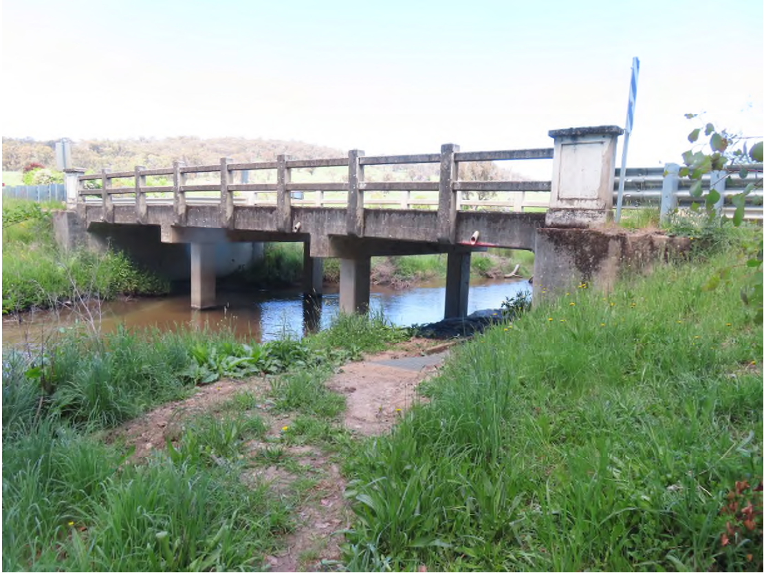
Photo 1. View from north side, west end. Note path under abutment nearest camera.
