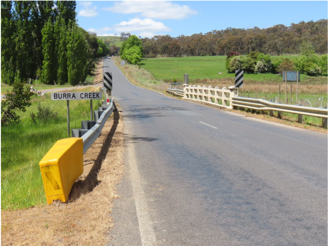
Photo 2. View of bridge from west end.
