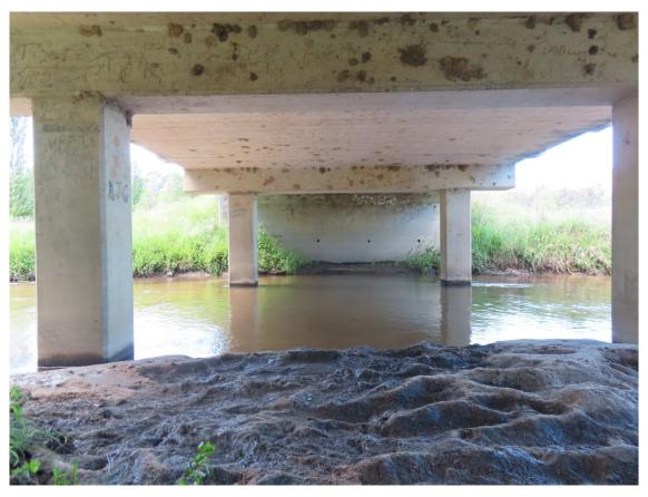
Photo 3. Underside of deck with pier columns and headstock. West span.
