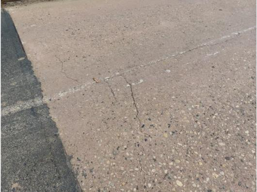
Photo 18. Transverse cracks in deck near east abutment.
