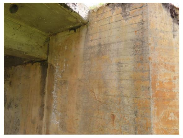
Photo 12. Typical crack in wingwall/abutment
