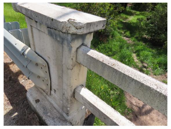
Photo 4. Minor damage to bridge rail post with some cracking.
