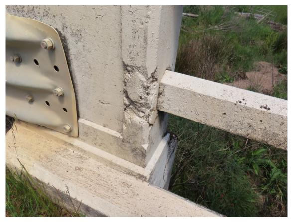
Photo 5. Minor damage to bridge rail post.
