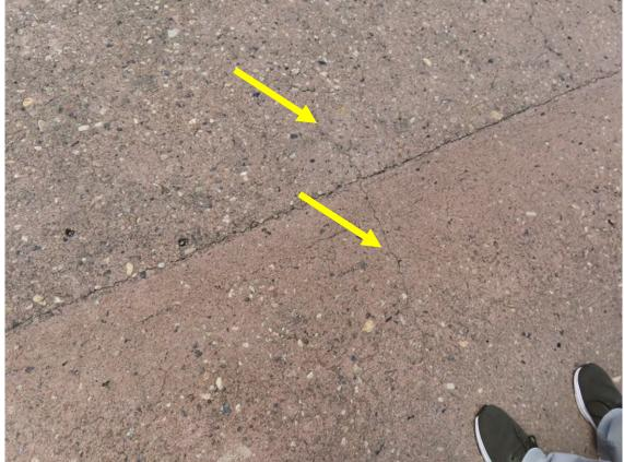
Photo 16. Transverse crack (arrowed) and longitudinal construction joint in deck
