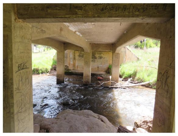
Photo 11. Underside of bridge. Note flood debris at pier.
