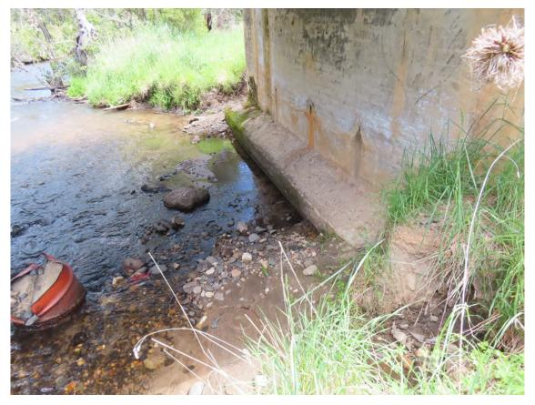
Photo 20. West abutment with slight erosion.
