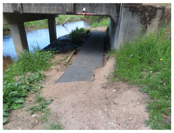
Photo 7. Track of composite mesh material under Tumbarumba abutment.
