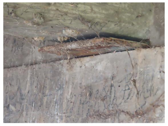
Photo 14. Tumbarumba (west) abutment. Centre beam bearing dislodged.
