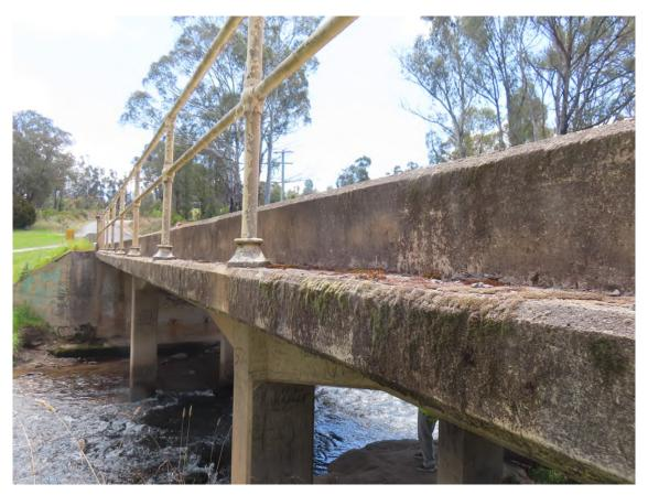
Photo 21. Side of bridge showing fixing arrangement for bridge railing.
