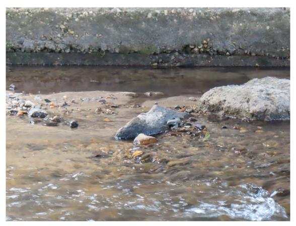
Photo 19. West span showing slight exposed footing under abutment.
